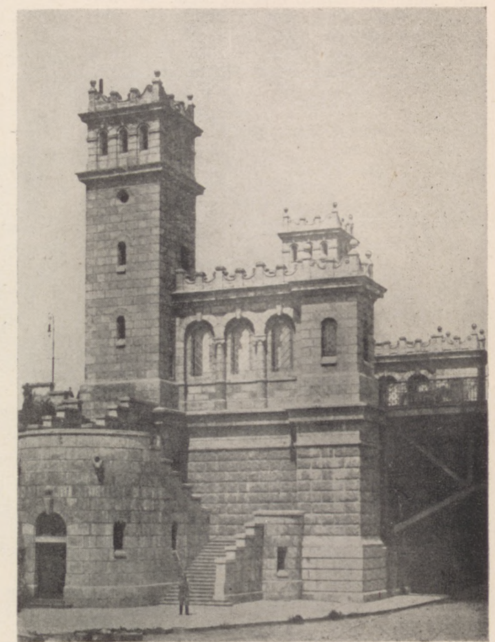
Gate tower, Joseph Poniatowski Bridge, Warsaw.
