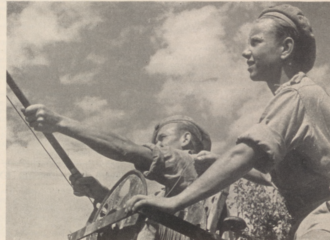
Polish signal corps men putting up telephone wires in Italy.
