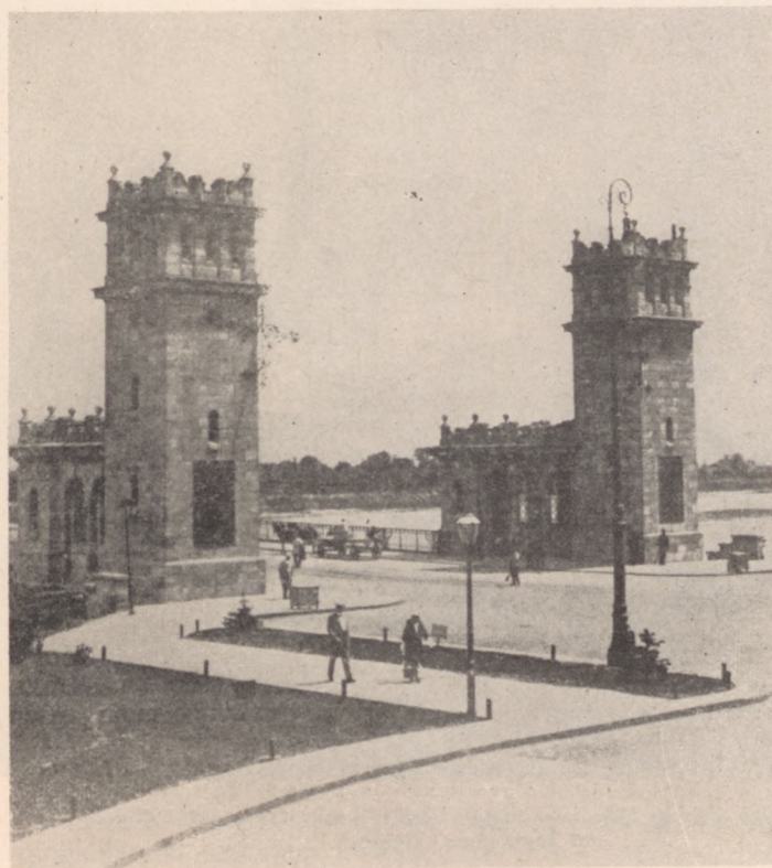
Approach to the Joseph Poniatowski Bridge, Warsaw.
