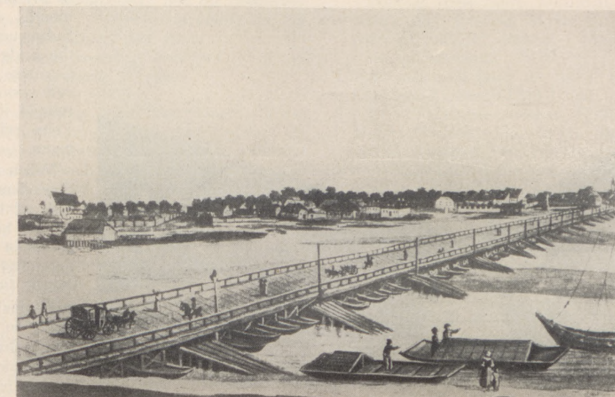
Floating bridge built at Warsaw by Adam Poninski in 1775. Water color by Vogel.
