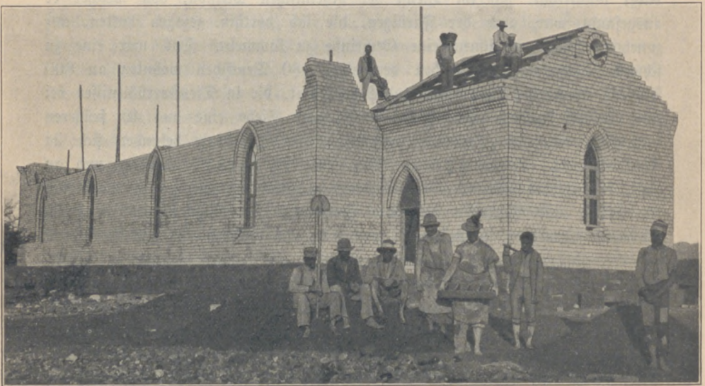
Kirchbau in Windhut.
