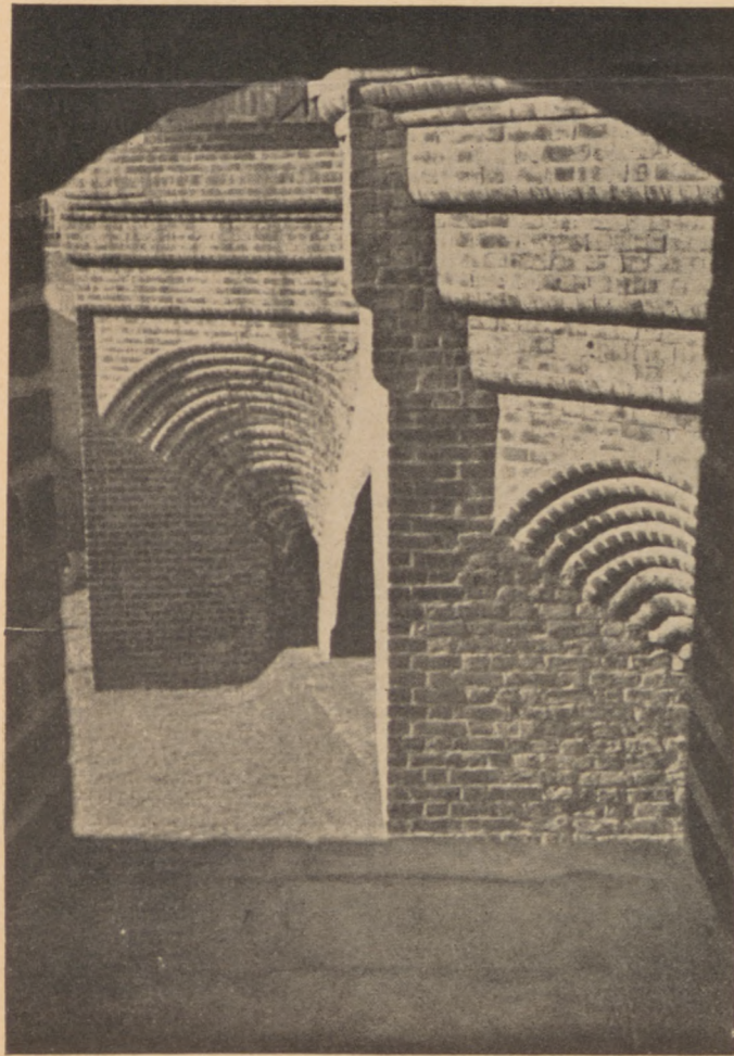
Restored fragment of old walls in Warsaw.
