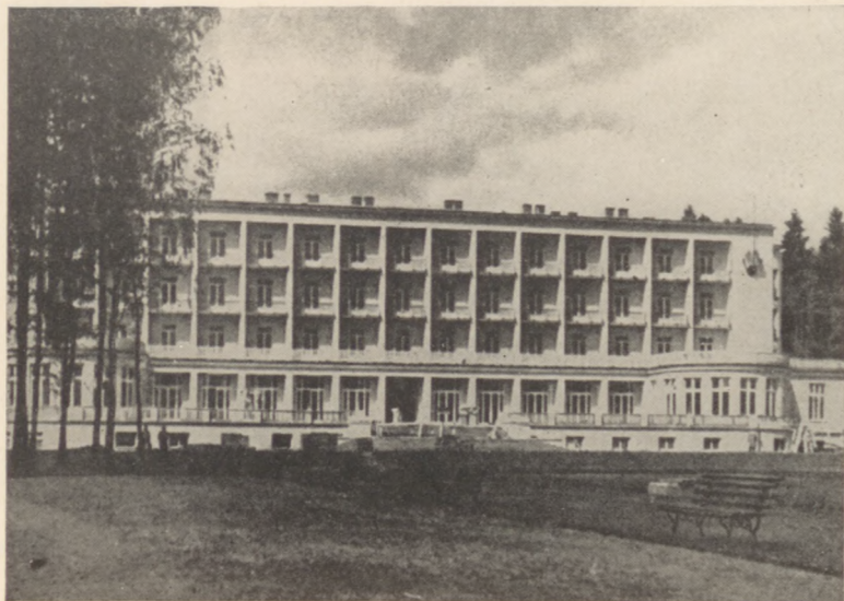
Sanatorium at Morszyn, Southeastern Poland.
