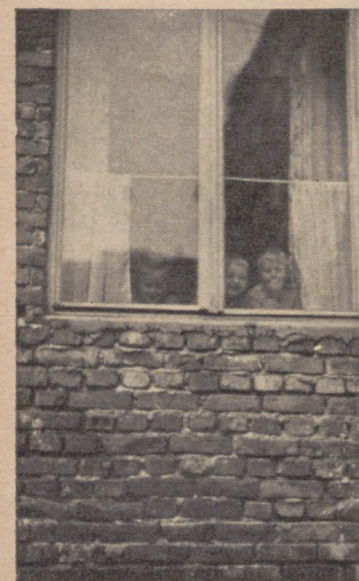
The brick has still to be faced but the flat is occupied
