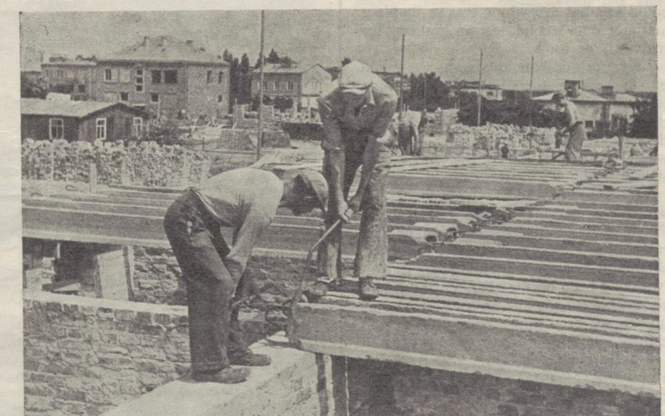
Laying prefabricated frames of reinforced concrete on the Mokotow site.
