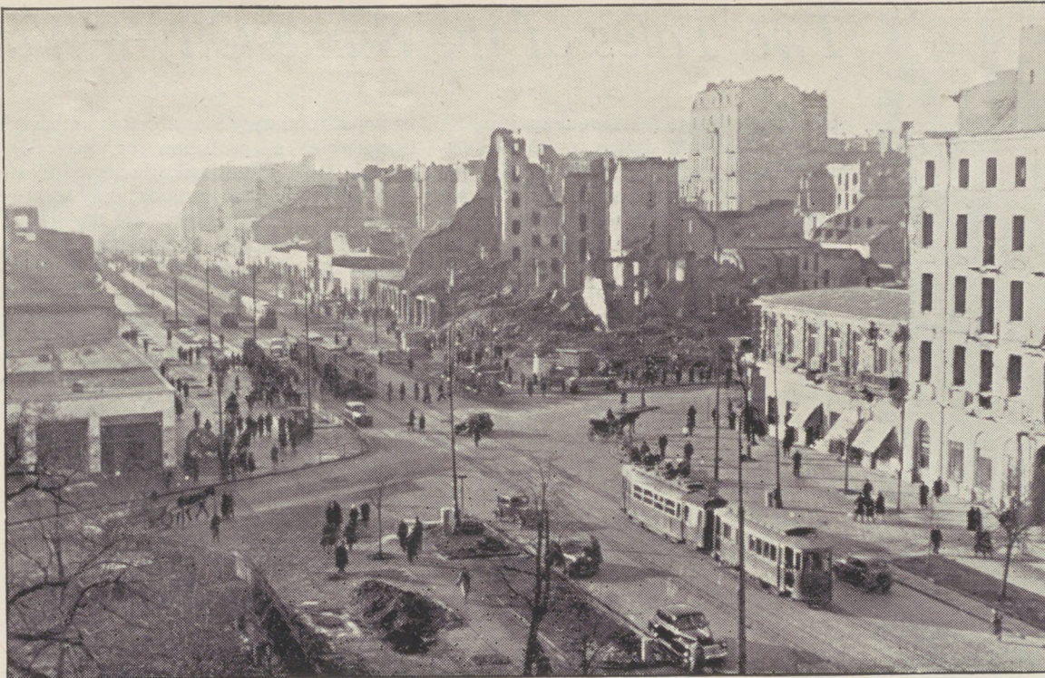
SPRING, 1948— Traffic flows freely through streets once choked with rubble.
