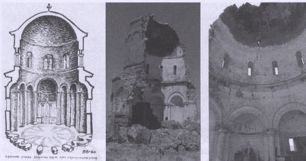
Fig. 8. Round Church rotunda: a - longitudinal section (reconstruction by Stefan Boyadjiev); b - Holy Savior at Ani - interior; c - Holy Savior at Ani -interior/exterior (photos by Yarus Ozkaya)
