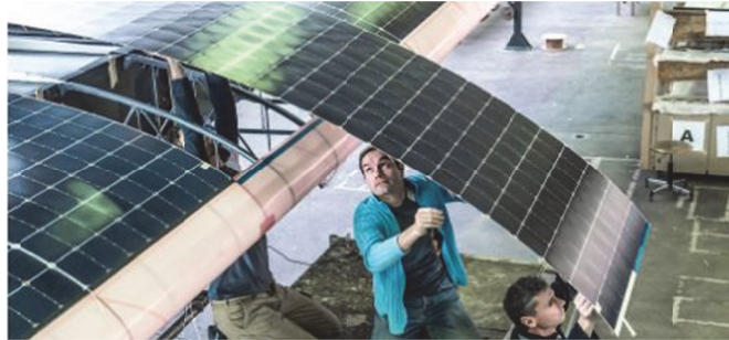
Fig. 14. Photovoltaic panels installation on Solar Impulse wings [11]
