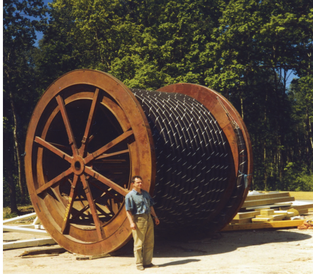
Fig. 3. 500 meters section of main cable ready for laying in the ground at the Polish side [own source]
