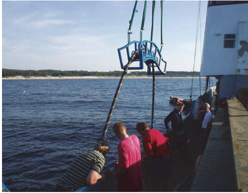
Fig. 5. Repair of the damaged return cable: a) the moment of taking out the cable from the water b) electrically damaged strands of a return cable [own source]
