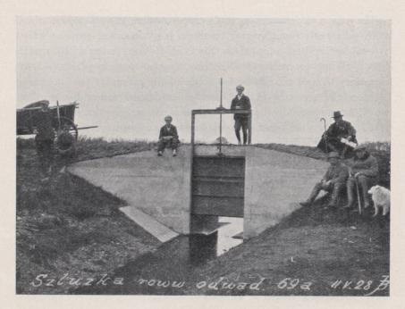
The lock, made of concrete and wood, controls the amount of water in the ditch — sometimes for drainage, sometimes for irrigation!
