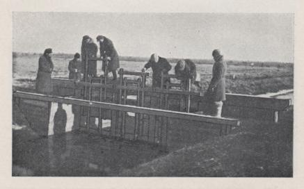
A lock in the main ditch on the land drained by the Experiment Station at Sarny.
