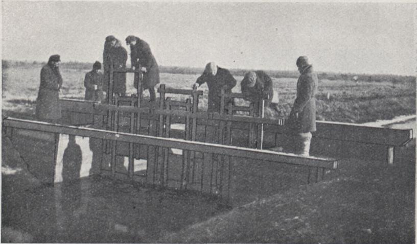
A lock in the main ditch on the land drained by the Experiment Station at Sarny.
