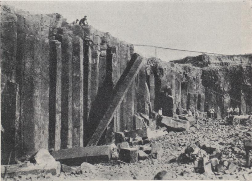
In the quarry at Janowa Dolina I watched a sixty-ton column of basalt fall into the pit, to be broken up, cut into blocks, and used in making new highroads.
